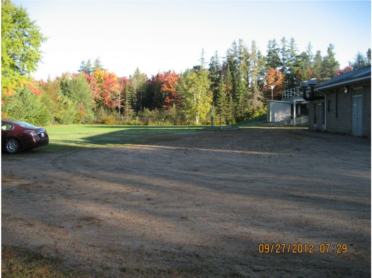
Photo: Chalk River WWTP vacant land available for expansion
